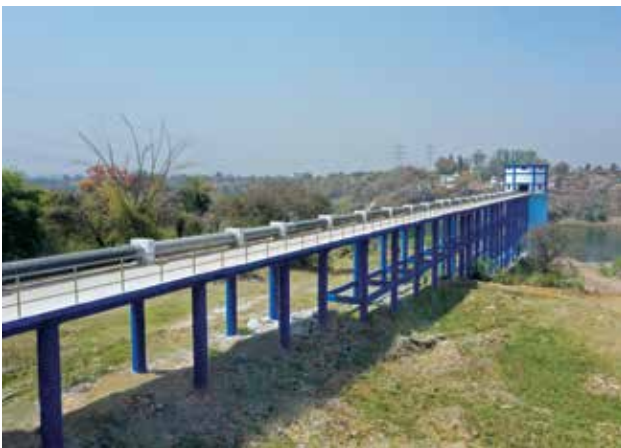
Intake well cum pump house at Bhedaghat Town, for Bhedaghat Water Supply Scheme, in Madhya Pradesh.
