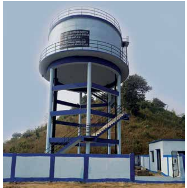
240 KL Overhead Tank staging 12 mtr at Village-Jajagarh, for Indwar-I Multivillage Rural Water Supply Scheme in Umariya and Katni District, in Madhya Pradesh.
