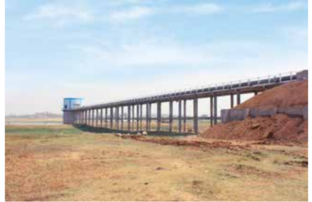
Intake Well cum Pump House with approach bridge in village -Jhal, for Indwar-I Multivillage Rural Water Supply Scheme in Umariya and Katni District, in Madhya Pradesh.
