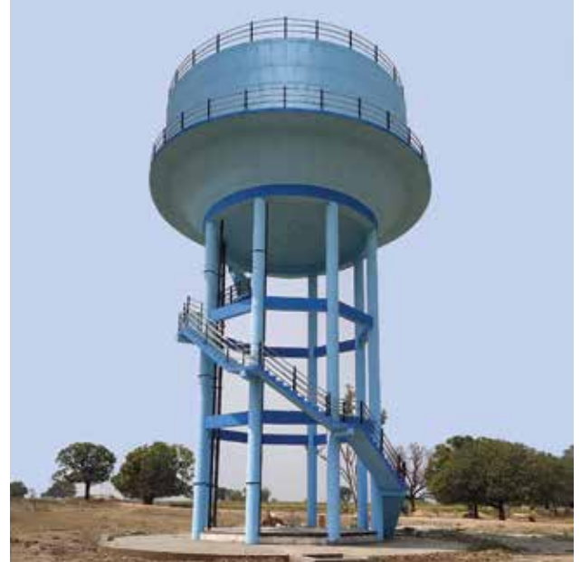
400 KL Overhead tank for Kandaila Multi village Rural Water Supply Scheme in Rewa district, in Madhya Pradesh.
