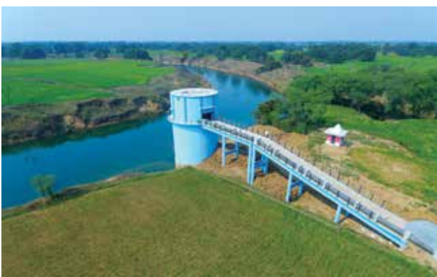
Intake well cum pump house for Kandaila Multi village Rural Water Supply Scheme in Rewa district, in Madhya Pradesh.
