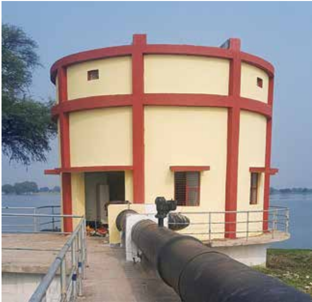
Intake well cum pump house, 8 Meter dia, 26 meter depth with ultimate capacity of 28.35 MLD with 520 meter approach bridge at Kolvi Village of Mandsaur project, in Madhya Pradesh.
