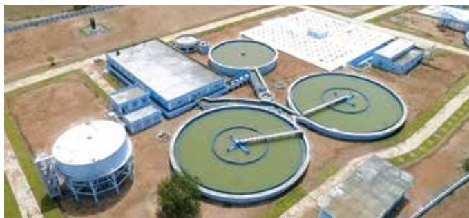
70 MLD Water Treatment Plant for Jurala (TDWSP) Project, in Telangana.
