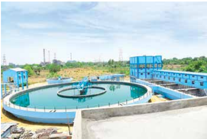
29 MLD Water Treatment Plant at Korba, in Chhattisgarh
