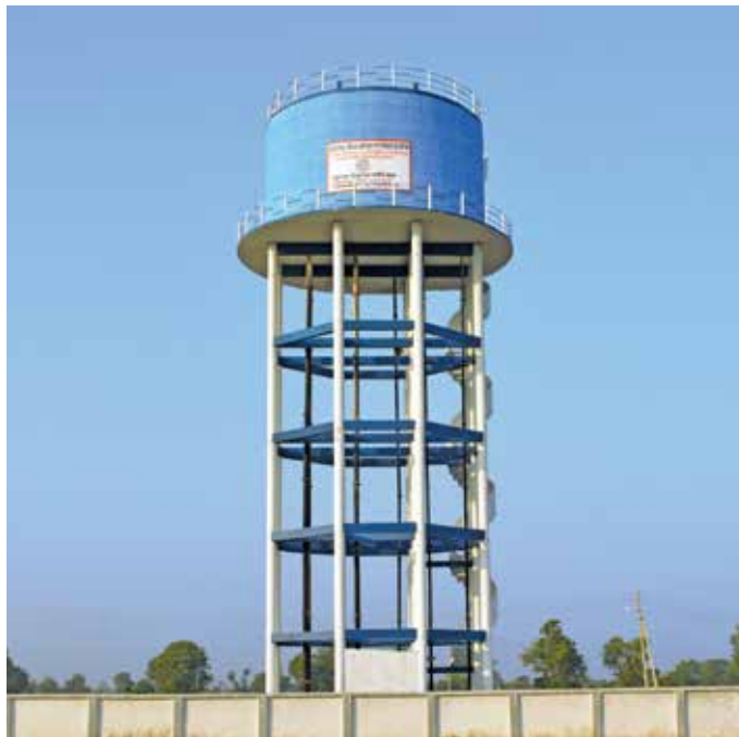
6.25 Lakh Litre Capacity Master Balancing Reservoir for Jalgaon Jamod Water Supply Scheme, in Maharashtra
