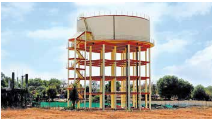
2,000 KL OHBR at Kushmonda for Guna Water Supply Project, in Madhya Pradesh.
