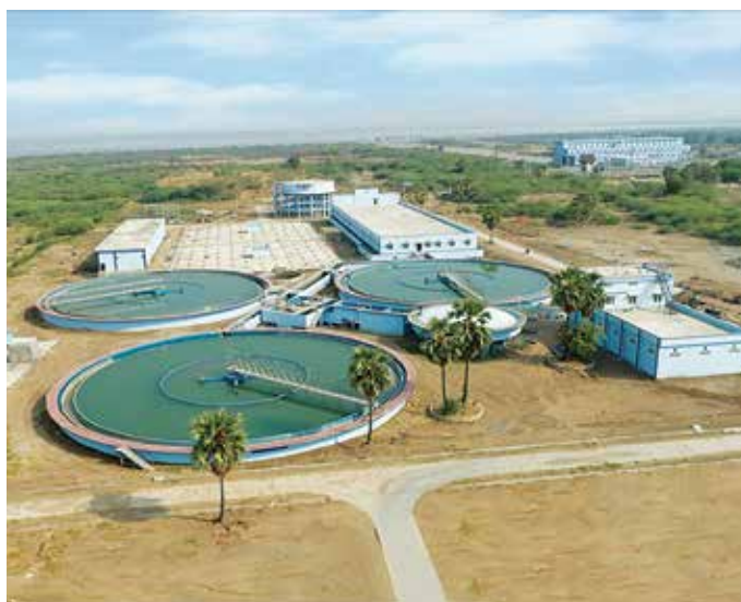
160 MLD Water Treatment Plant at Murmur village, Yellampally, Peddapali, Ramagundam for TDWSP Circle, Karimnagar, in Telangana.
