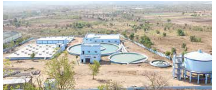
40 MLD Water Treatment Plat at Mallannagutta for Balkonda (TDWSP)Project, in Telangana.
