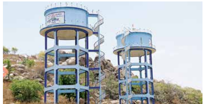
90 KL OHSRs at Balkonda for intra-village works for Balkonda (TDWSP) Project, in Telangana.
