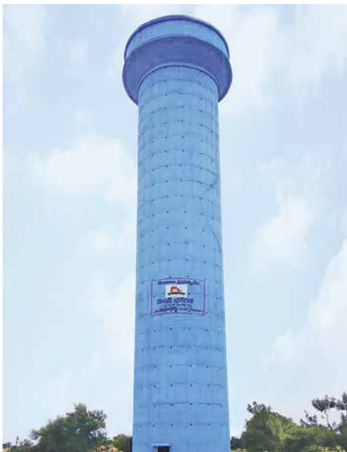
90 KL x 30 Meter Staging OHBR at Mallamdoddi for Jurala (TDWSP) Project, in Telangana.
