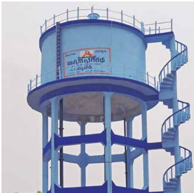
120 KL x 12 Meter Staging OHBR at Jammichedu for Jurala (TDWSP) Project, in Telangana.
