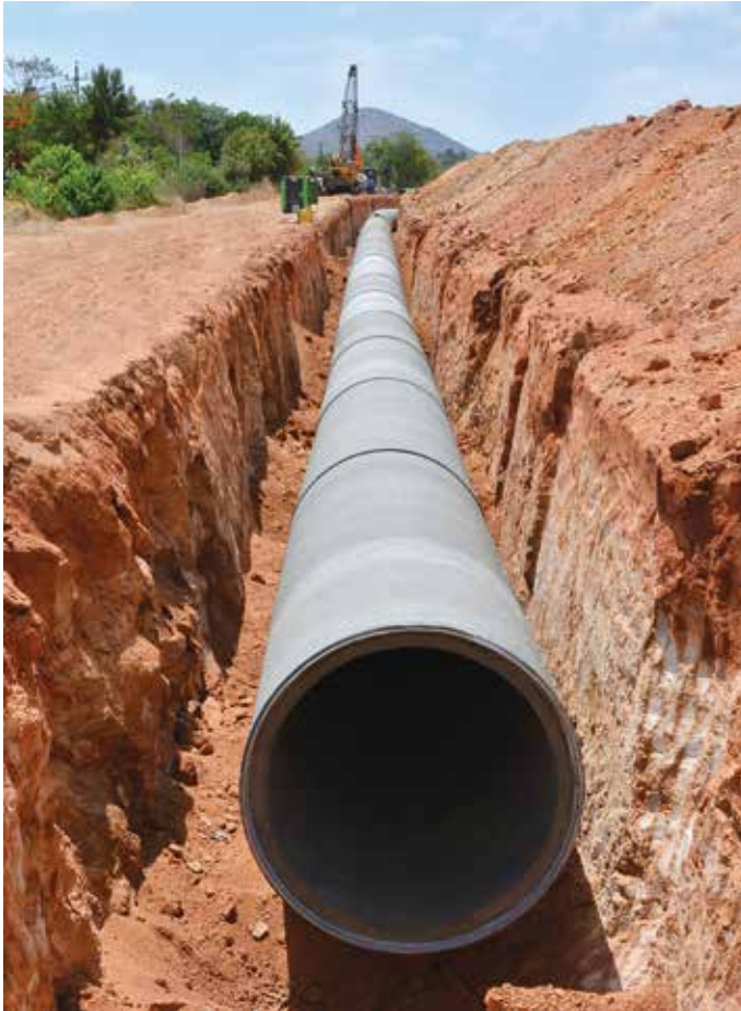
800 mm dia MS pipeline laying at Jahazpur Project, in Rajasthan.
