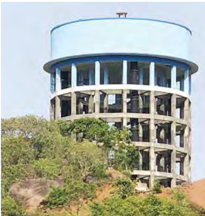
1000 KL OHBR at Manikbhandar for Balkonda Project in Telangana
