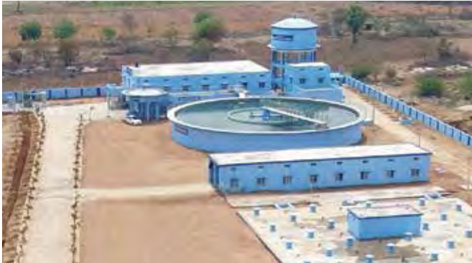
20 MLD Water Treatment Plant for CPWS Scheme to Thungathurthy Project, in Telangana
