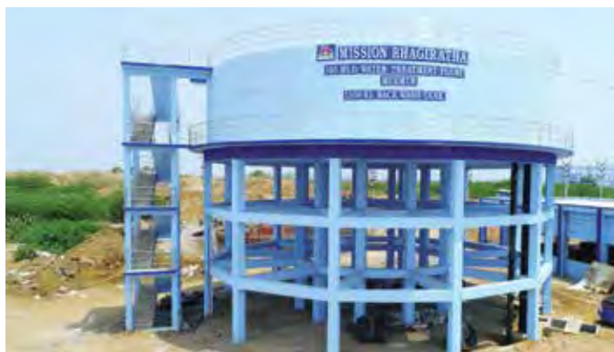
1200 KL back wash tank at Murmur for Karimnagar TDWSP Project in Telangana
