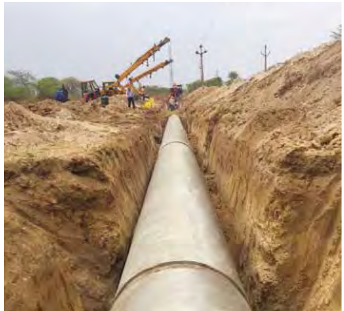
1500 mm dia PCCP pipeline laying for Balkonda Project, in Telangana
