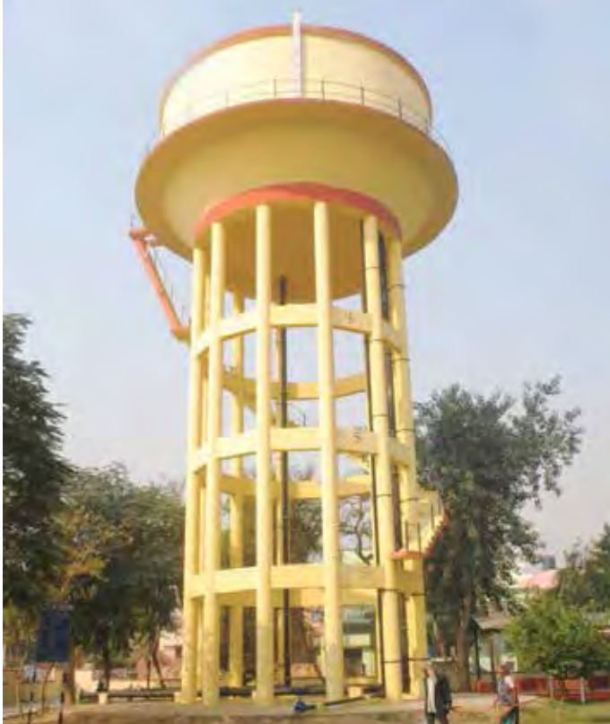
400 KL OHSR for Urban Water Supply Scheme Alwar, in Rajasthan
