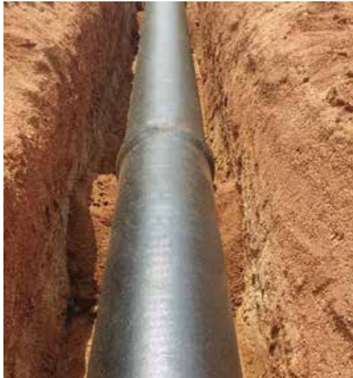
1000 mm dia DI K-7 pipeline at Jurala Segment for Jurala (TDWSP) Project, in Telangana
