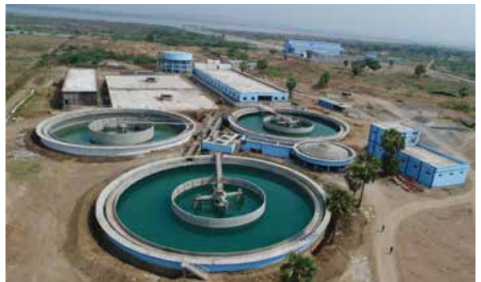
160 MLD Water Treatment Plant at Murmur Village Yellampally for Karimnagar (TDWSP) Project, in Telangana.
