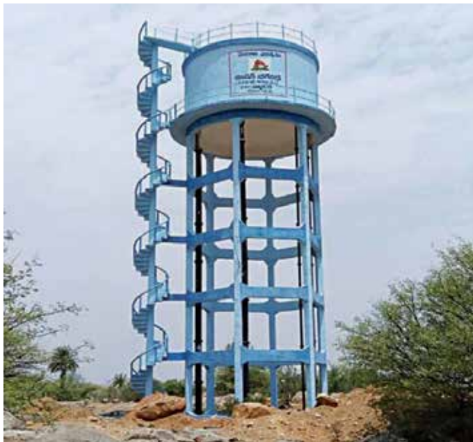
90 KL x 15 Mtr staging OHBR at Maldakal for Jurala (TDWSP) Project, in Telangana
