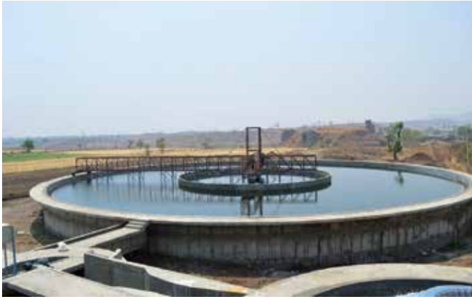
Clariflocculator for 31 MLD water treatment plant at Jalgaon Jamod Water Supply Scheme, in Maharashtra
