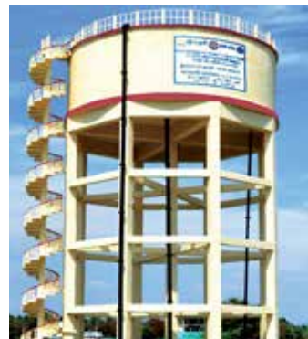
3 Lakh Litre Capacity 16 Meters Height Service Reservoir for Palladam Water Supply Project in Tamilnadu
