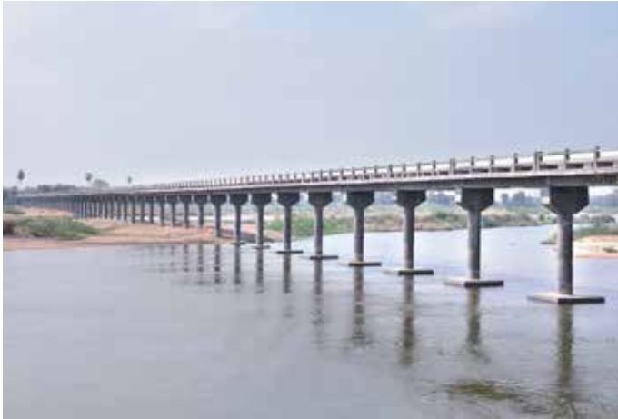
580 meters long Foot Bridge at Cauvery River carrying 711 mm dia M.S. Pipeline for CWSS to Pudukottai in Tamilnadu.
