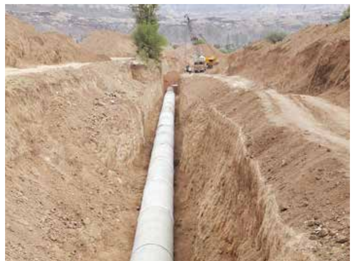
1500 mm dia PCC pipeline laying for Chilhwadi pipeline project in Maharashtra
