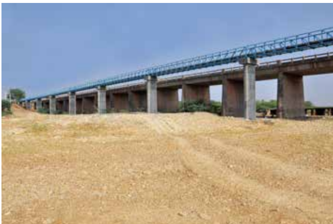
500 mm dia DI pipeline on bridge over Sugileru river at Badvel Water Supply Scheme in Andhra Pradesh
