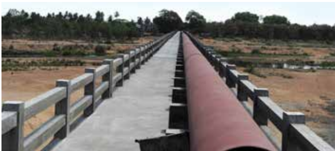
360 Mtrs length foot bridge at River Kollidam for 700 mm dia MS Pipeline at CWSS to Pudukottai, Tamilnadu
