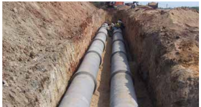
900 mm dia PSC pipeline laying for IFFCO Kisan SEZ Nellore, Andhra Pradesh
