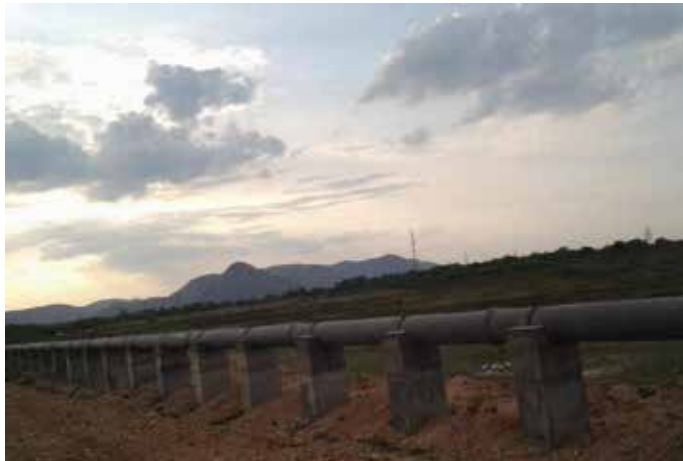
500 mm dia DI pipeline for Badvel Municipality Water Supply (Package-I), Andhra Pradesh
