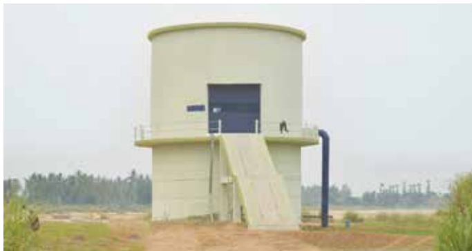
Collection well at Head Water Works at River Nagavali For Rajam Water Supply Improvement Scheme, Andhra Pradesh
