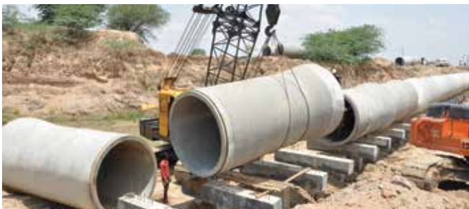
2000 mm dia PSC pipes laying for Pulikanuma L.I.Scheme, Andhra Pradesh
