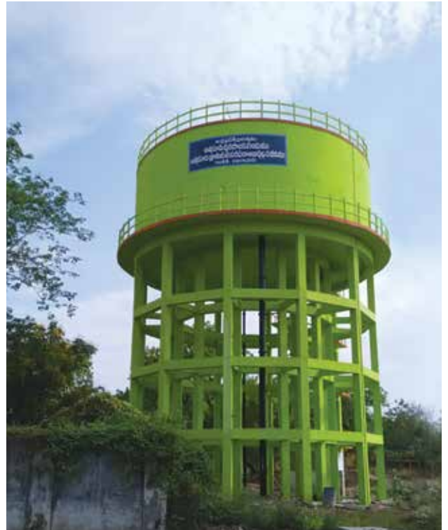
7 Lakh litre capacity Elevated Storage Reservoir for Atmakur Project, Andhra Pradesh
