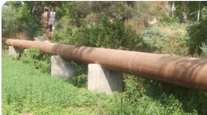
711 mm dia MS Pipeline for Sangamner Water Supply Scheme, Maharashtra
