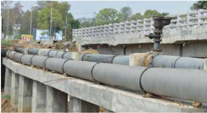
600 mm dia DI pipeline laying for Chhindwara Water supply Scheme, Madhya Pradesh
