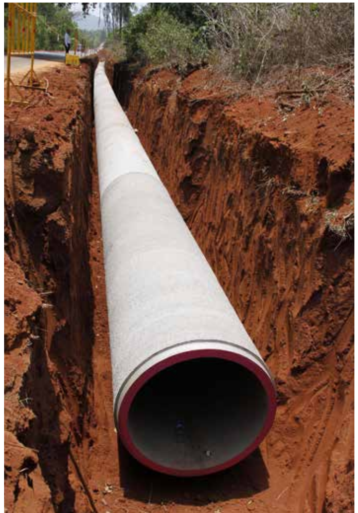
1200 mm dia PCC pipes laying for Tillari Water Supply Scheme, Maharashtra
