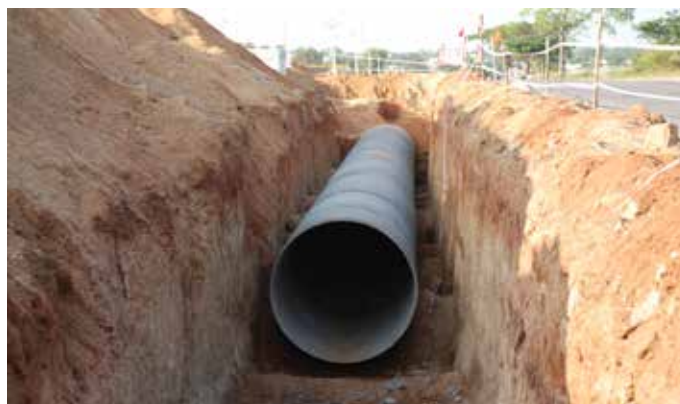
2200 mm dia MS pipeline for Krishna Drinking Water Supply Project Package-IV Phase-III, Telangana
