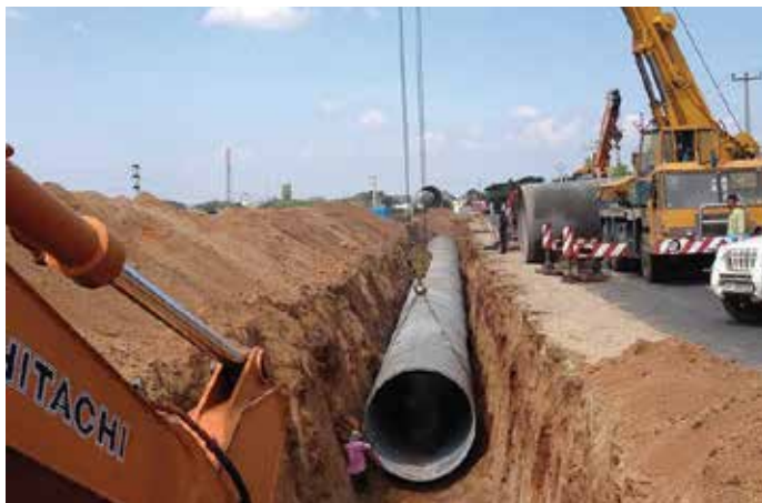
2200 mm dia MS Pipes for Krishna Drinking Water Supply Project Phase-III Package-IV, Andhra Pradesh
