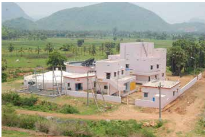
Water treatment plant for CPWS Scheme to Yelleshwaram, Prathipadu, Samkhavaram & Kirlampudi, Andhra Pradesh
