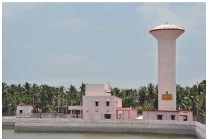
90,000 Ltr. Overhead Balancing Reservoir with Intake well cum-pump house of 4.5 Mtrs Dia for Amalapuram Water Supply Scheme, Andhra Pradesh
