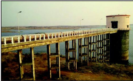
Intakewell with Pump House & footbridge for Anantpur EPC Project
