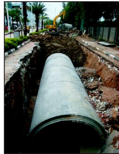
2400 mm dia RCC NP3 class pipe for Bangalore water supply and Sewerage Board Bangalore.
