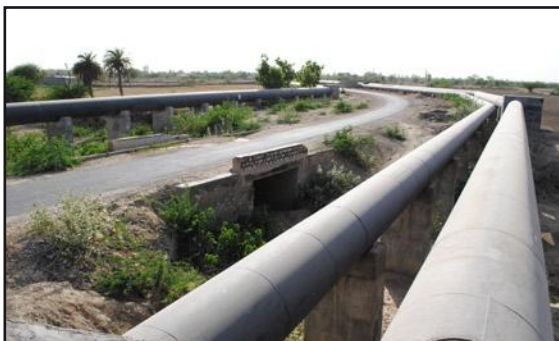
Ajmer Water Supply Scheme involving MS pipe line in Rajasthan State
